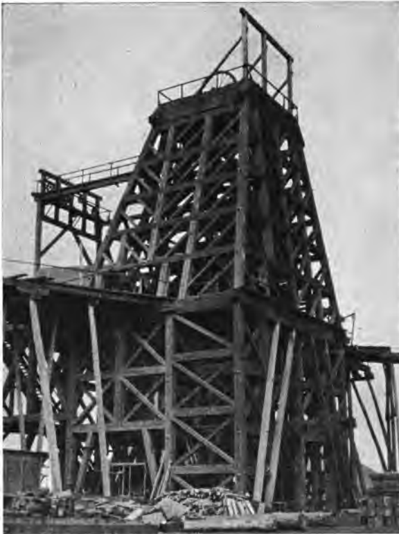
Fig. 2. Wooden Head Frame, East Norrie Mine, Oliver Iron Mining Co., Ironwood, Mich.
